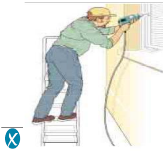
Incorrect – steps side on to work activity
