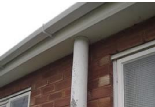
Asbestos cement drainage pipe (downpipe)
