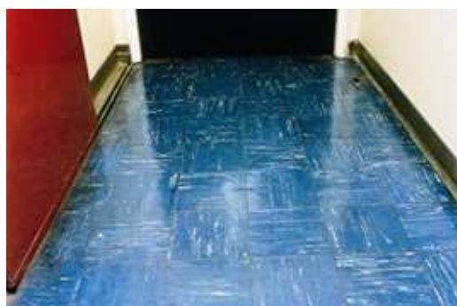
Asbestos containing floor tiles in a corridor
