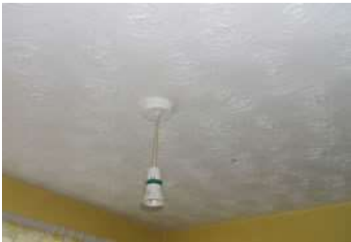
Asbestos textured coating
