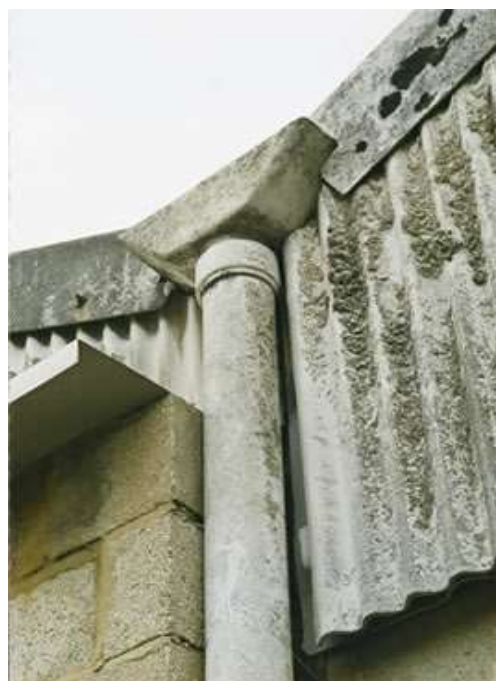
Asbestos cement downpipe, hopper and profile sheet
