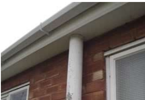
Asbestos cement drainage pipe (downpipe)
