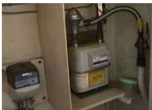
Asbestos panelling around a gas meter
