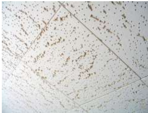
Asbestos containing ceiling tiles
