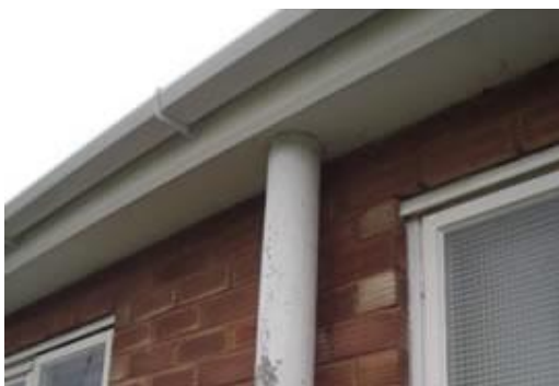
Asbestos cement drainage pipe (downpipe)
