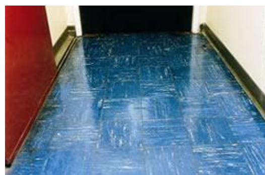
Asbestos containing floor tiles in a corridor
