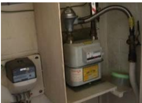
Asbestos panelling around a gas meter
