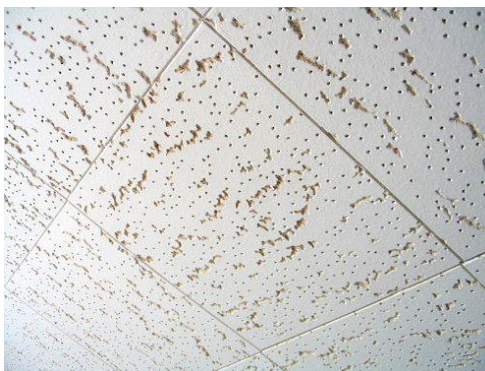
Asbestos containing ceiling tiles
