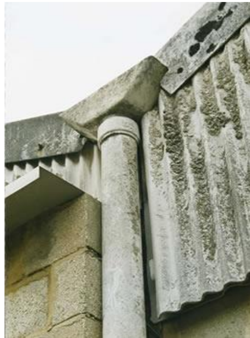
Asbestos cement downpipe, hopper and profile sheet
