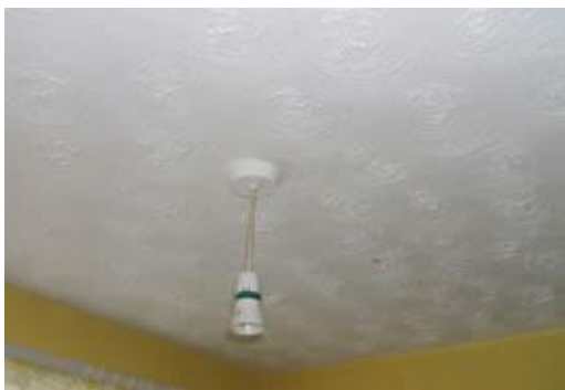
Asbestos textured coating
