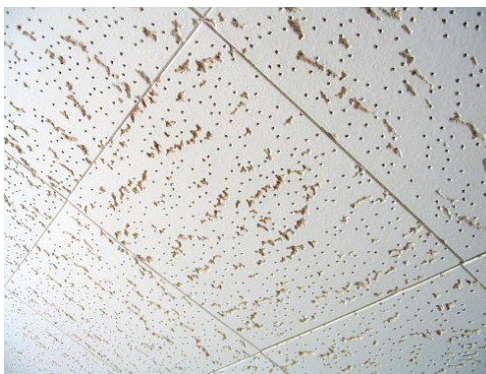
Asbestos containing ceiling tiles
