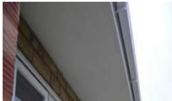
Pieces of Asbestos Insulating Board (AIB)
