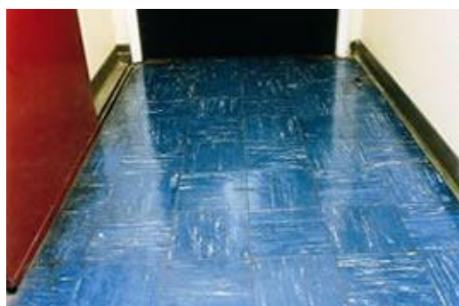
Asbestos containing floor tiles in a corridor
