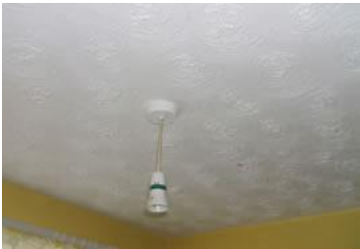
Asbestos textured coating
