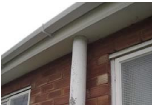
Asbestos cement drainage pipe (downpipe)
