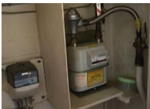
Asbestos panelling around a gas meter
