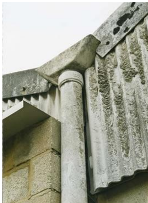
Asbestos cement downpipe, hopper and profile sheet
