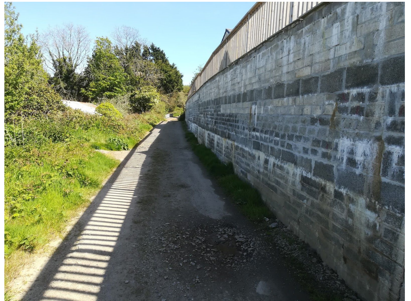
12. Concrete retaining wall separating new development from Tolskithy valley
