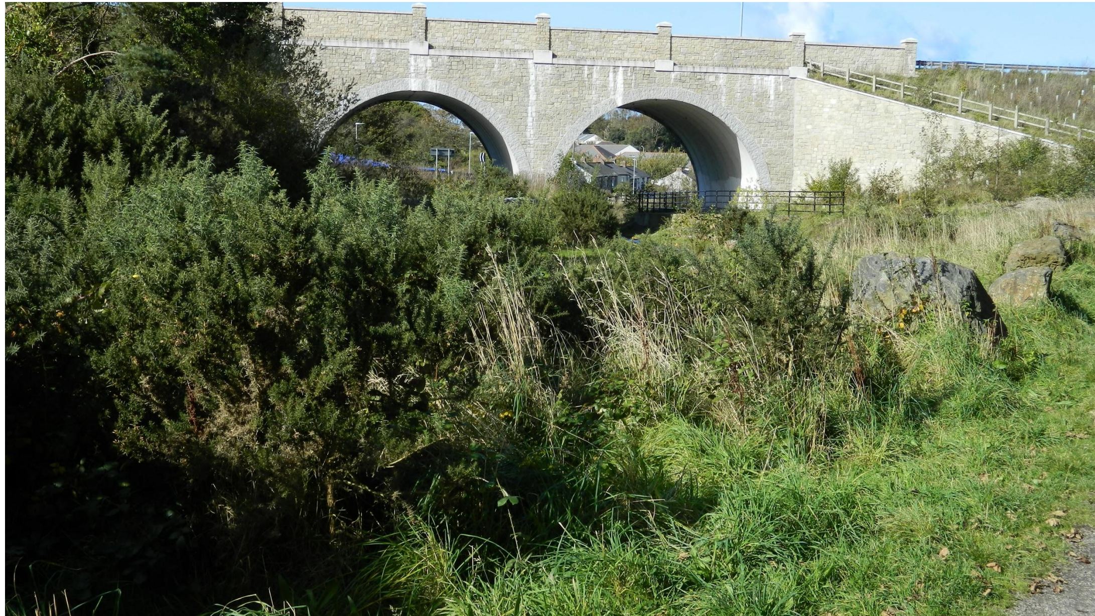
18. The new bridge at Kerrier Way.
