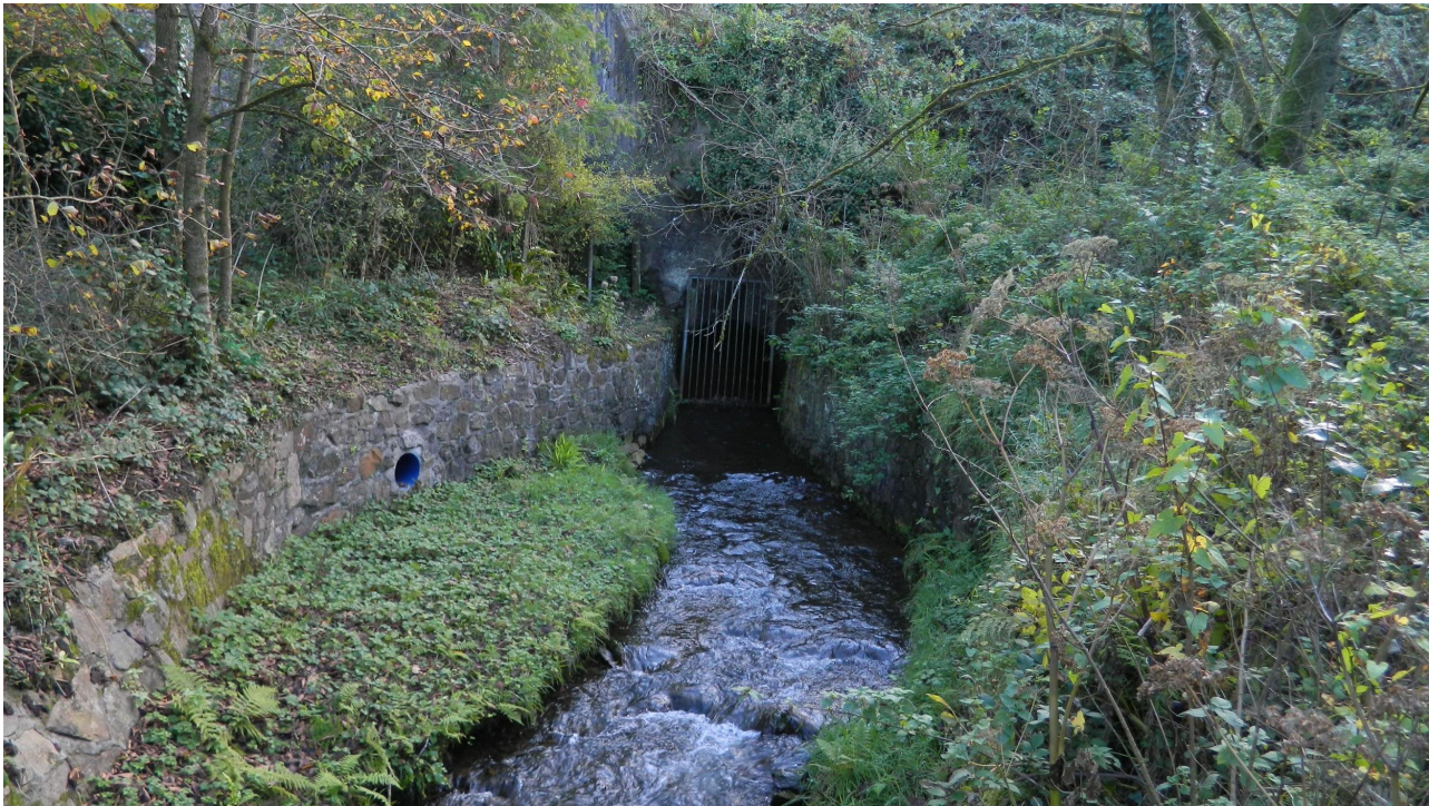
3. River emerging from railway embankment
